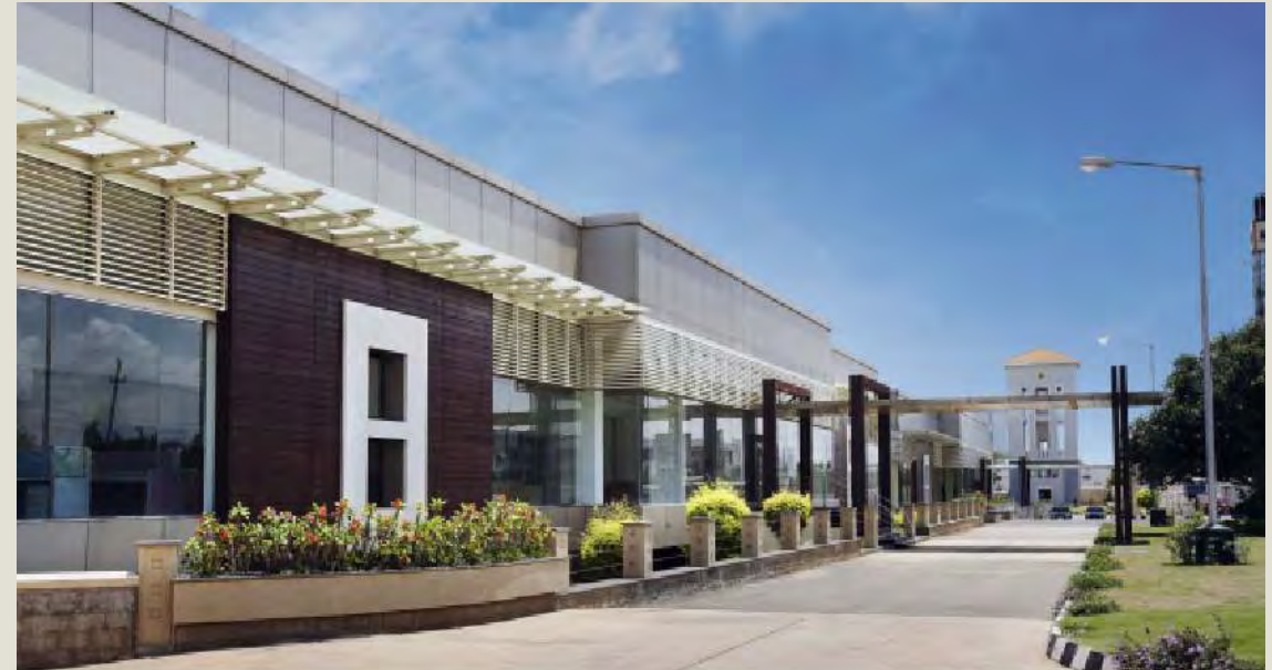
Sobha Manufacturing Unit
